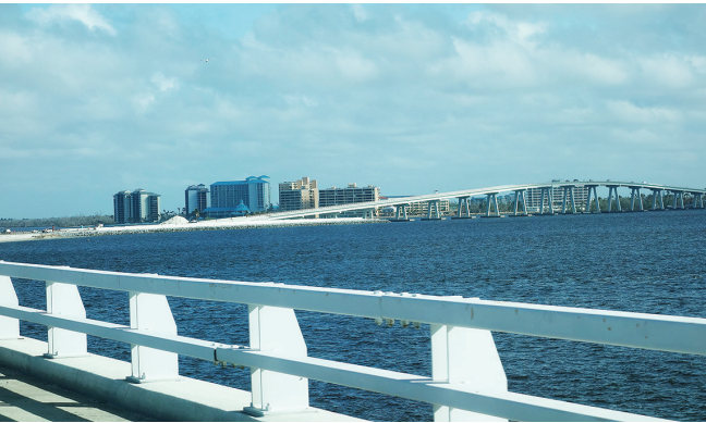
The newly rebuilt causeway is two feet higher so the boats can go underneath it. Before the hurricane damaged the structure, there was a drawbridge that opened and you had to wait for the boats to pass through. Higher is better so you do not have to stop on the bridge and wait. It is still three miles long.
