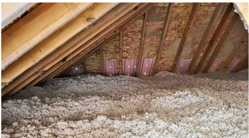
Insulation & Air Sealing
